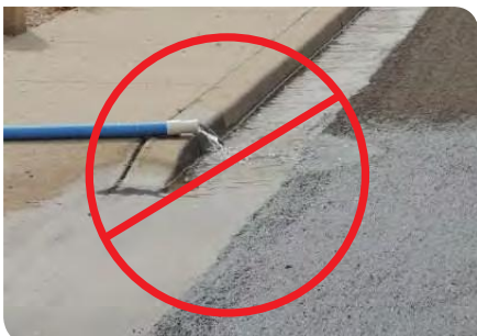
Improper draining of pool backwash onto impervious surface leading to a storm sewer intake. (Cape Water Harvest)
